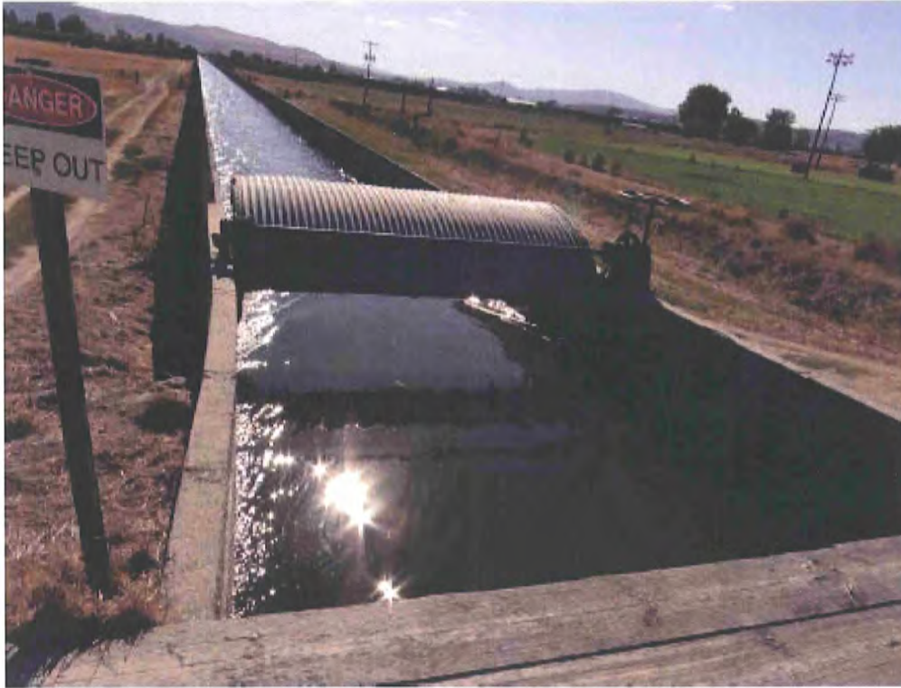
(Photo 6) Beginning of the north end of the C Flume looking south
