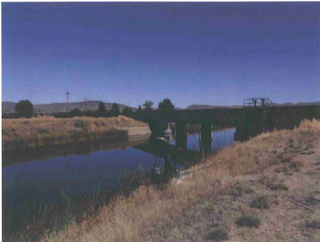
(Photo 3) C Flume Crossing the LRDC looking northeast
