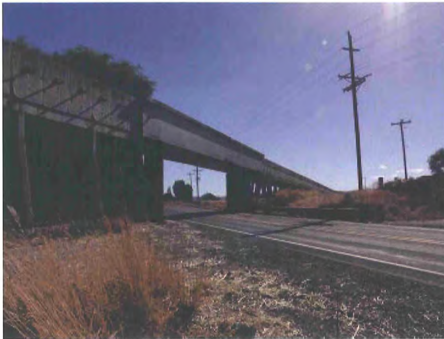
(Photo 5) C Flume crossing over Highway 39
