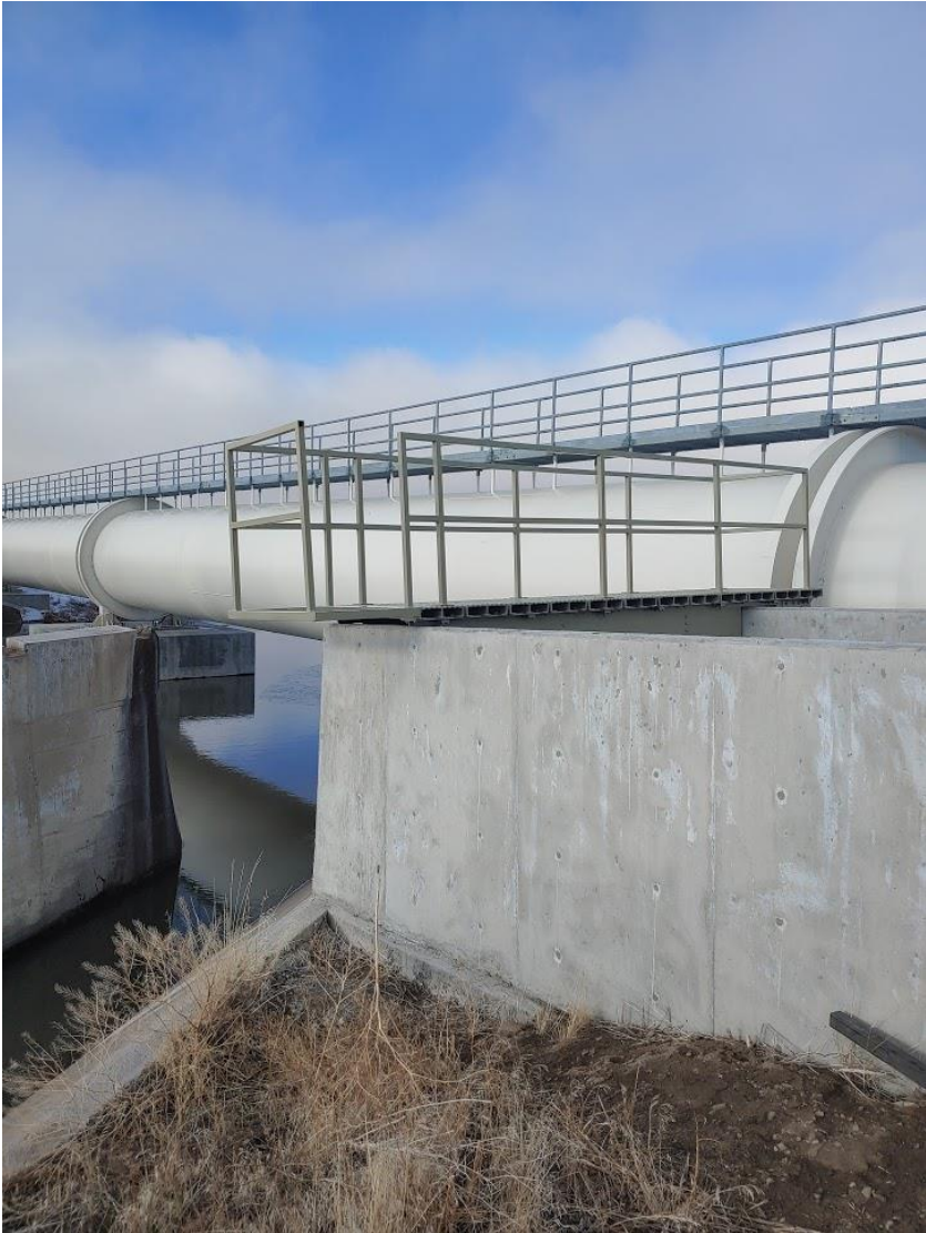
C –Siphon Spill Catwalk Installation
