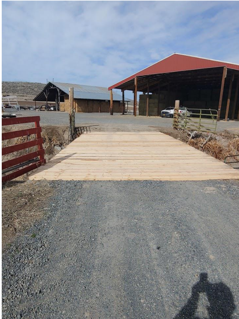
Dave Wilson Bridge Repair C-4
